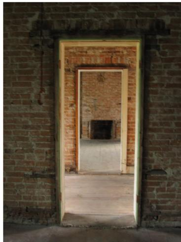
1820s floorplan of the Stephenson House, Tolman's consists of two front rooms separated by an entryway. With the third room connected to one of the front rooms. The house's walls are two courses of brick thick, while the foundation is three courses thick. It is believed that the floorplan of the house consists of the entryway/hallway which opens to the bedroom on one
